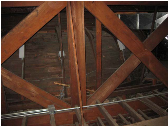
Photo #59: Attic above council chamber– note lack of insulation
