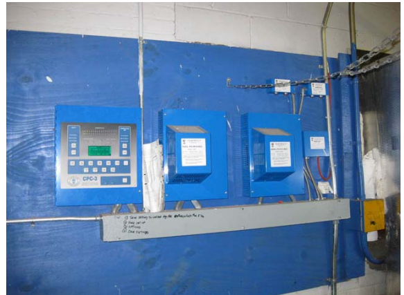
Photo #10: Combustion air VFDs
