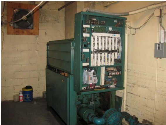
Photo #47: Elevator controller and machine
