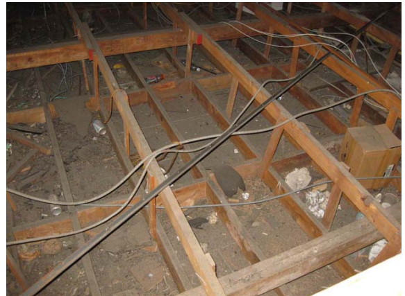
Photo #58: Attic – note lack of insulation
