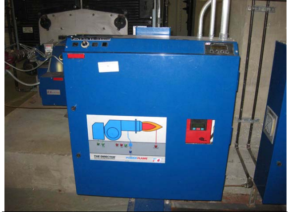
Photo #14: Burner controller
