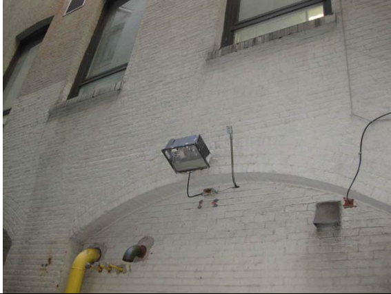
Photo #43: Exterior metal halide fixture
