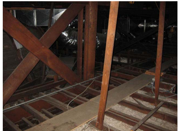
Photo #60: Attic above council chamber– note lack of insulation
