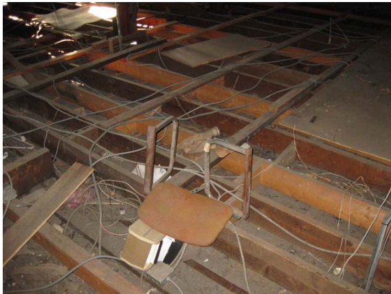
Photo #57: Attic – note lack of insulation
