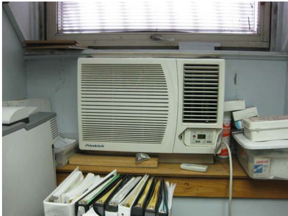
Photo #21: Typical window air conditioning unit
