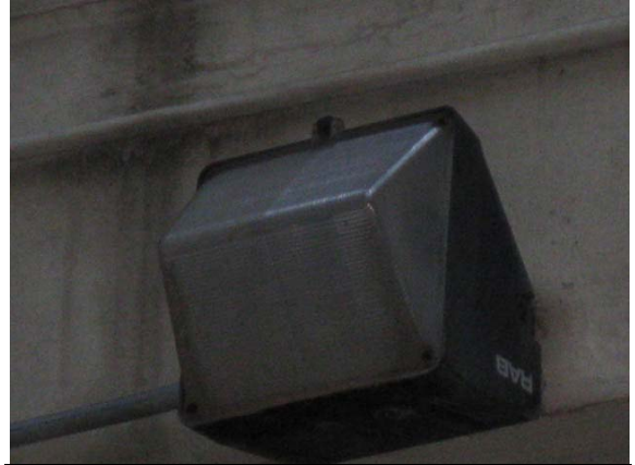
Photo #44: Exterior high pressure sodium fixture
