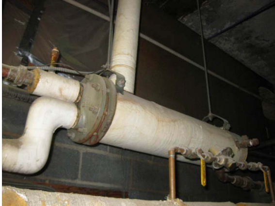
Photo #19: Basement hot water loop heat exchanger
