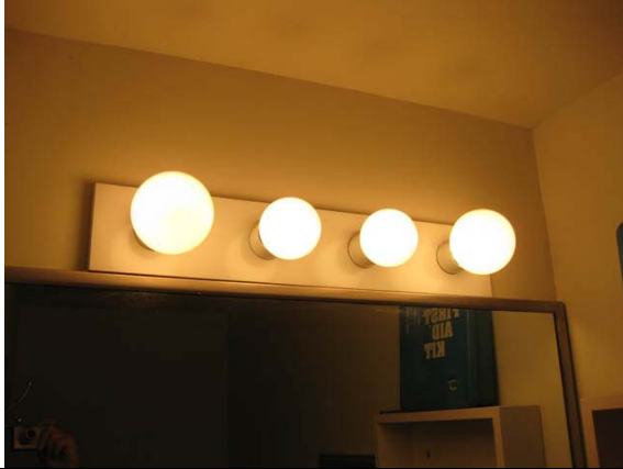
Photo #37: Office bathroom incandescent lighting
