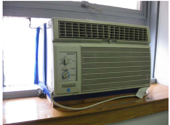
Photo #52: Typical window air conditioning configuration
