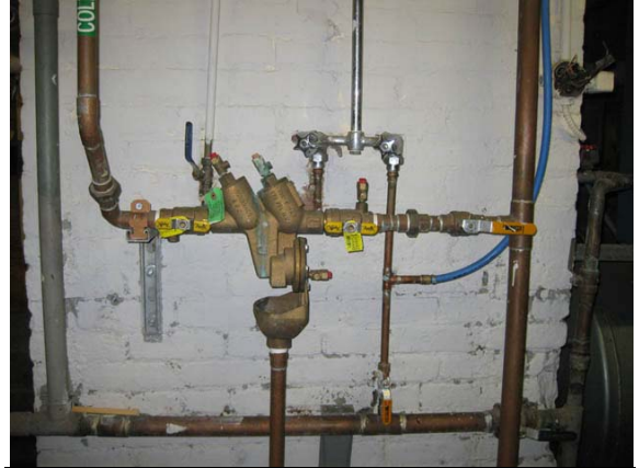
Photo #32: Heating system makeup backflow preventer
