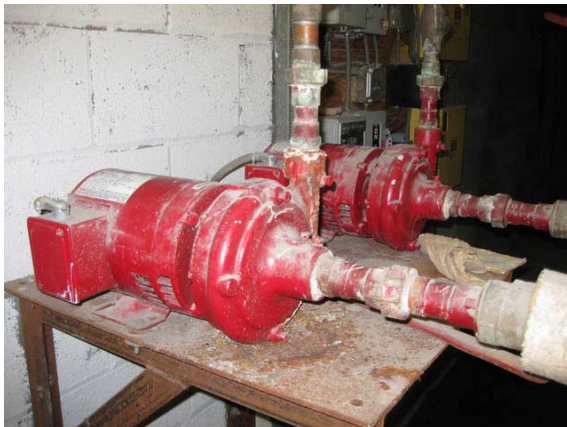
Photo #17: Basement hot water circulation pumps
