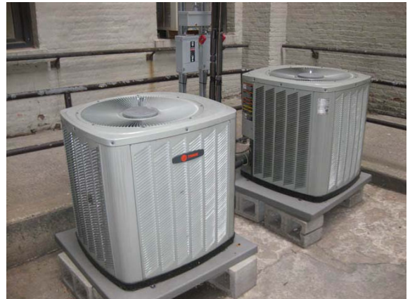
Photo #22: Computer room condensers
