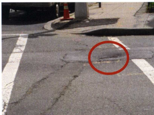
Reset PSE&G gas valve box on Ocean Avenue crosswalk to make flush with surrounding pavement to eliminate tripping hazard.
