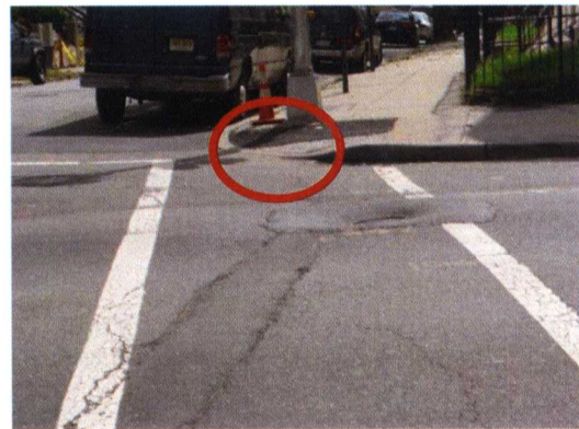
Provide detectable warning strips at all curb ramps at the intersection.
